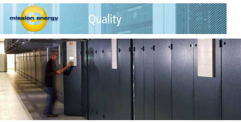
STULZ CyberAir 3 allows for both central and distributed arrangement of air conditioning units. Every unit has its own intelligence. Up to 20 units work together in the system network.
